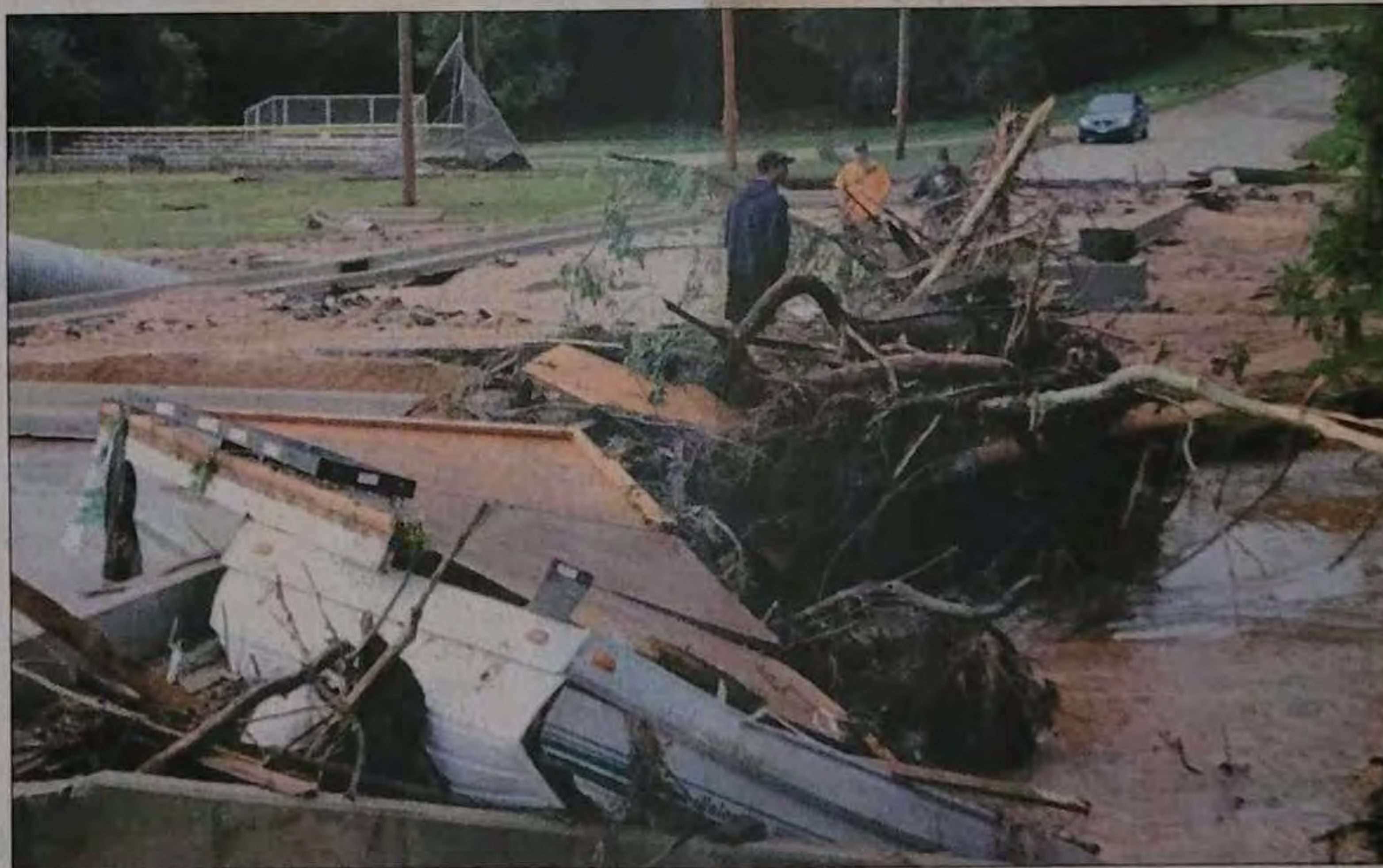
Debris piles up against Old Highway H, causing flood waters to surge through toward Waynesville Middle School and Slaughter Field. PHOTO CREDIT PAUL HACKBARTH
